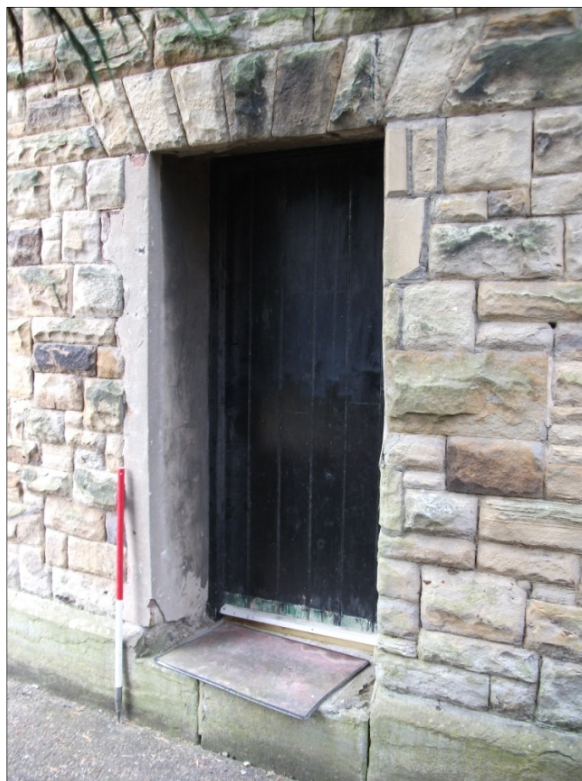
Fig 20: Doorway within gable on the Bothy's eastern elevation, looking SW.
