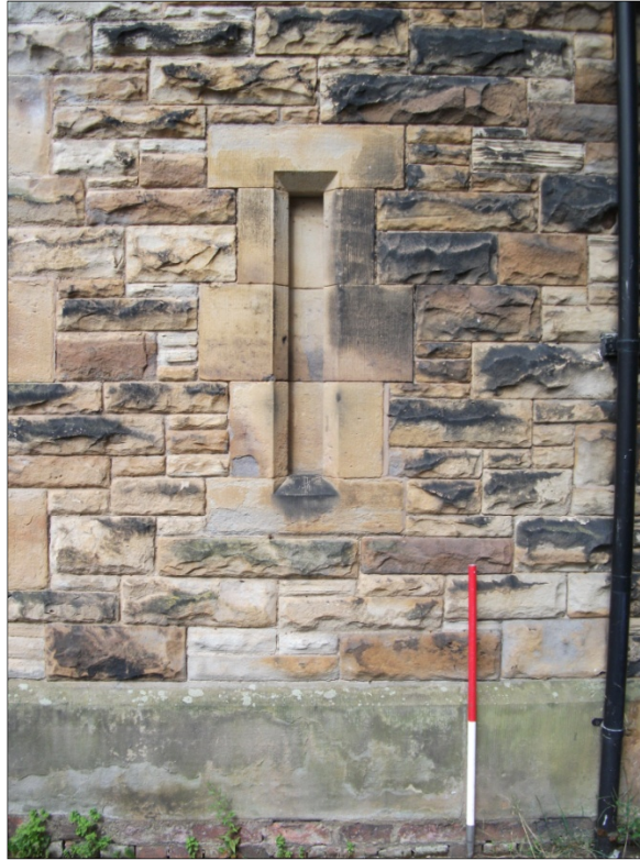
Fig 19: Blocked window at southern end of Bothy's eastern elevation, looking W.
