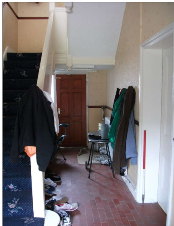
Fig 26: Southern and western walls of the Entrance Hall (G4), looking S.
