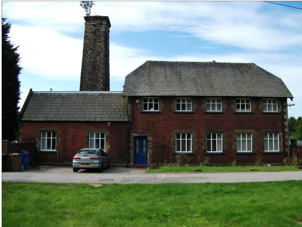
Fig 7: North elevation of Bothy, looking S.
