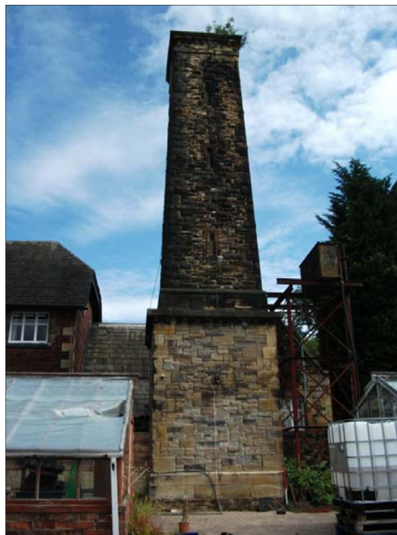
Fig 16: View of the south face of the stone chimney, which abuts the southern elevation of the Bothy, looking N.
