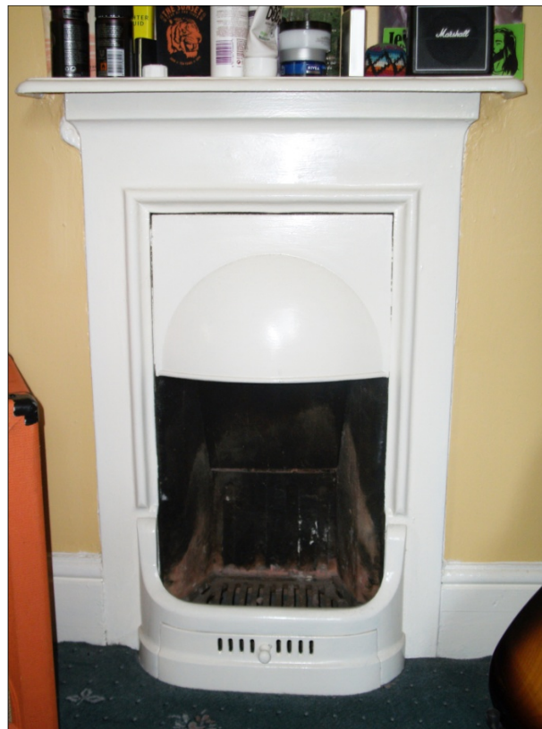
Fig 42: Detail of Fireplace within south-east corner of Bedroom 4 (F5), looking SE.
