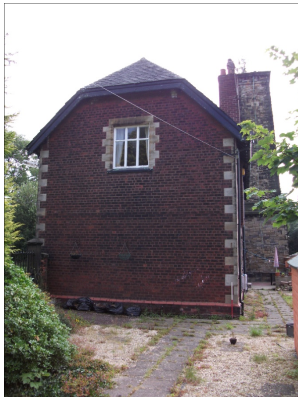
Fig 10: West elevation of the Bothy, looking NE.
