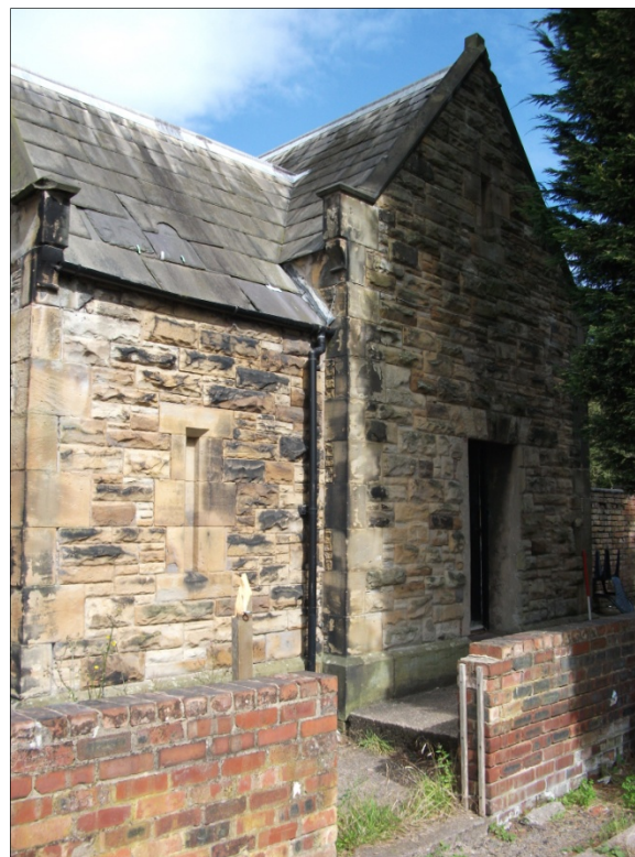
Fig 18: Eastern elevation of the Bothy, looking NW.
