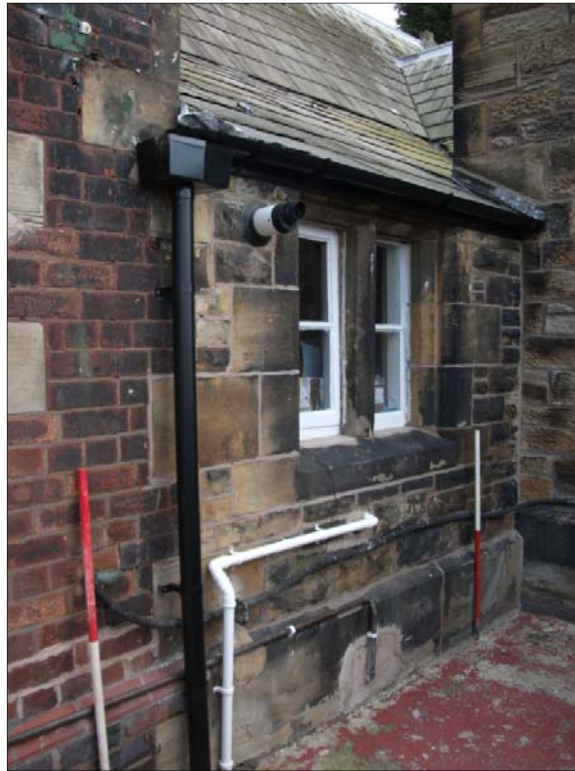
Fig 15: View of stone mullioned window on Bothy's southern elevation, looking NE.
