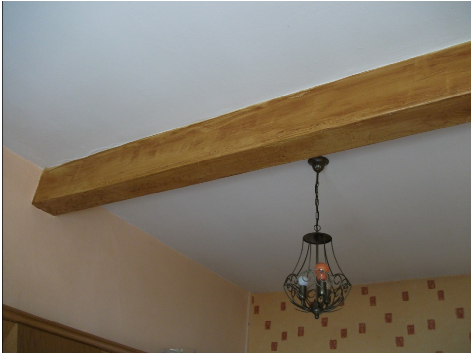
Fig 31: Detail of beam on Kitchen (G6) ceiling, looking NW.
