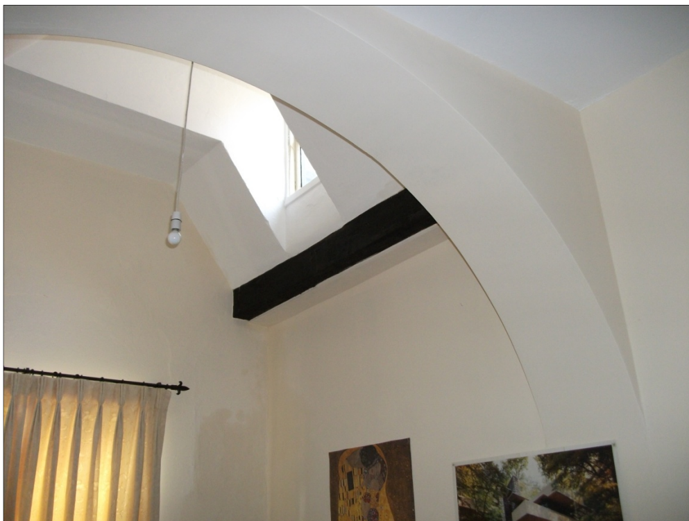
Fig 22: Detail of ceiling in south-west corner of Bedroom 1 (G1), looking SW.
