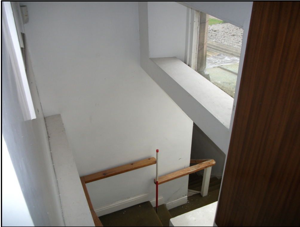
Figure 36 - View of the Upper Stairwell (F7). Looking north-west
