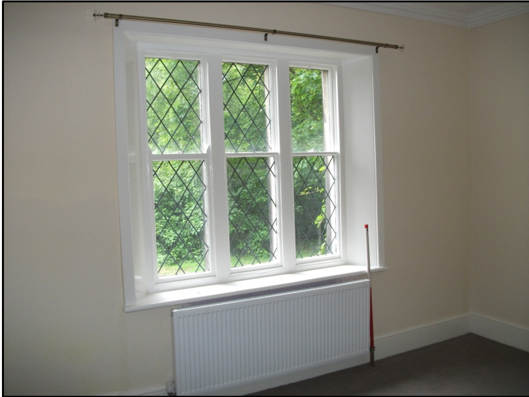
Figure 20 - Detail of the stone mullion window on the southern wall of the Dining Room (G4). Looking south-west
