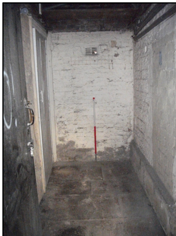
Figure 27 - View of the Privy Corridor (G12). Looking east
