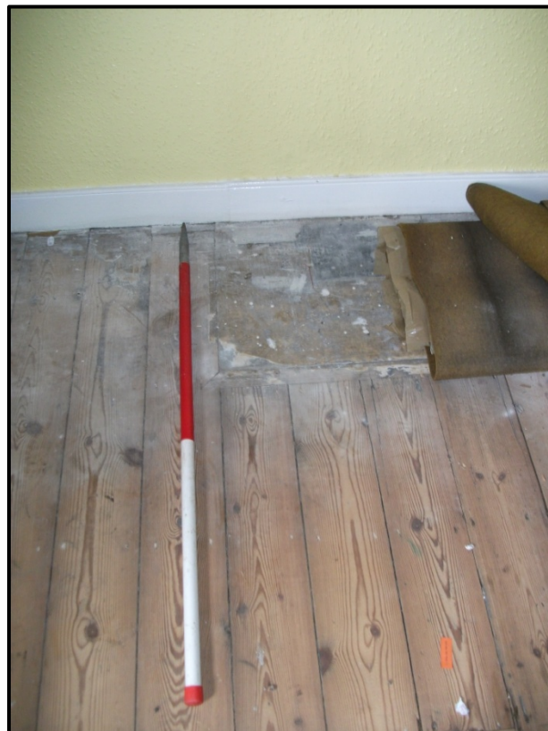
Figure 33 - Detail of blocked fireplace in western wall of the South Bedroom (F4). Looking west
