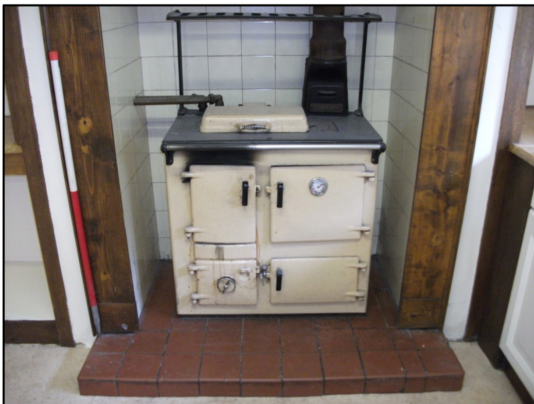
Figure 25 - Detail of Aga, abutting the north wall of the Kitchen (G10). Looking north-east
