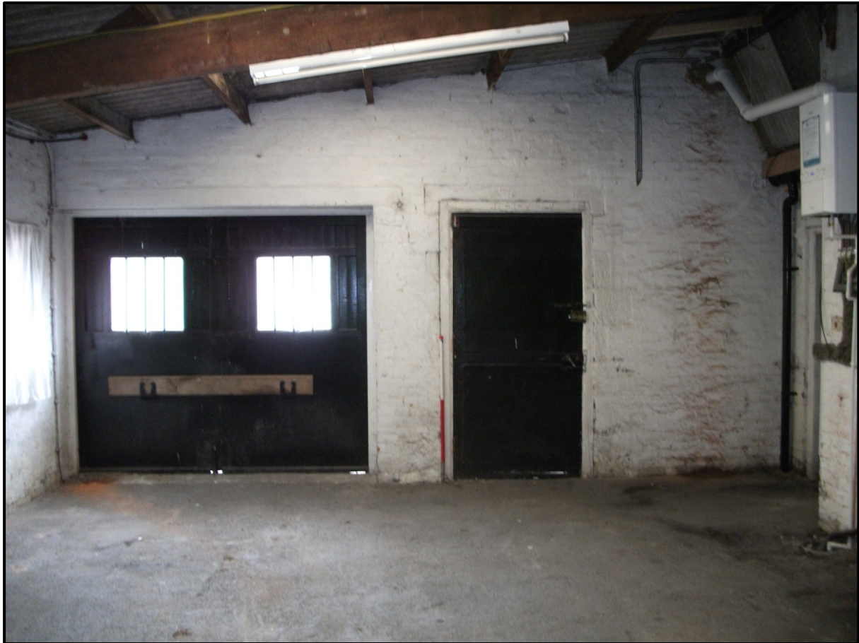
Figure 26 - View of the northern wall of the Garage (G11). Looking north-east
