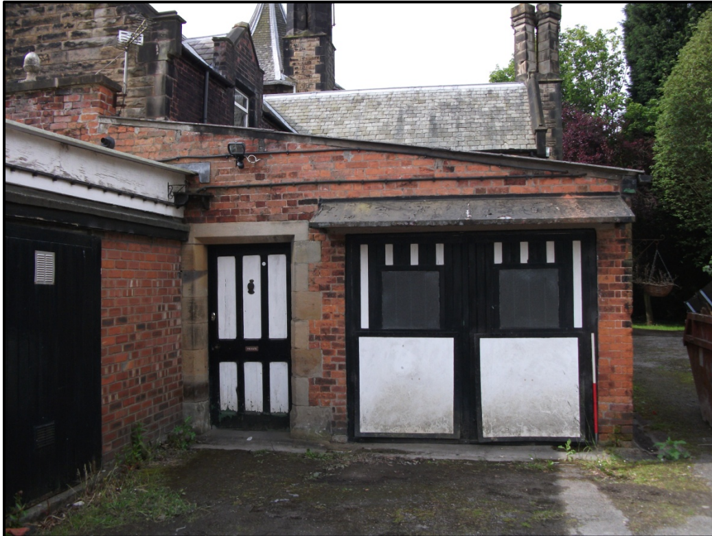
Figure 12 – View of the entrance ways into the garage at the northern elevation of the Garden Cottage. Looking south-west
