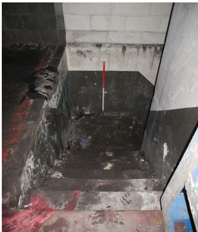
Figure 27: Shot taken of eastern stairwell S3 taken from corridor F4 on the first floor. Looking east.
