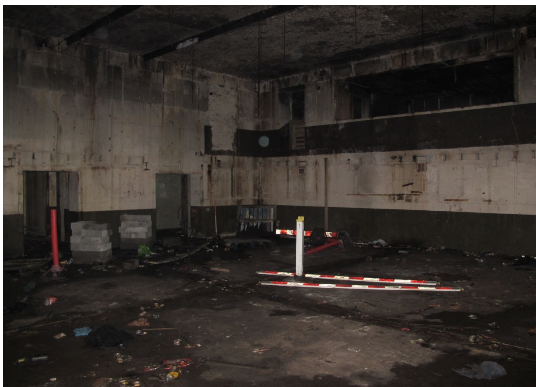
Figure 12: General shot of the main operations room G4 showing its western access points. The shot also shows the viewing gallery F5 on the first floor. Looking north-west.
