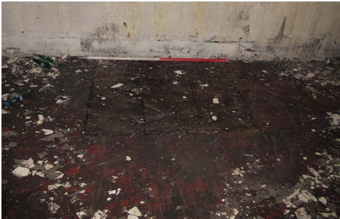
Figure 31: Detail of blocked southern stairwell S1 in room F1. The wooden hatch marks the location where the stairs would have risen to from corridor G1 on the ground floor.
