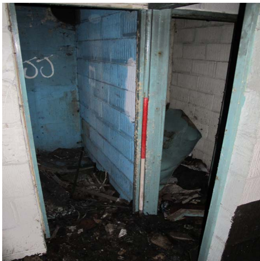
Figure 39: General shot of the breeze block toilet block in north-eastern room F6. Looking northeast.
