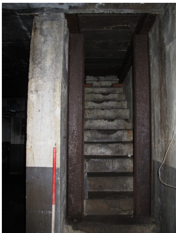
Figure 26: Detail of stairwell S1 which rose from corridor G1 to room F1 on the first floor. Access to F1 was found to be blocked by a wooden hatch built into the floor of F1.
