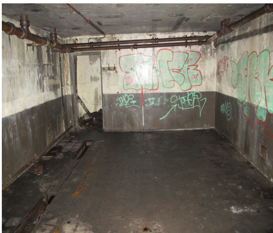
Figure 16: General shot of room G8, showing doorway leading to staircase S4. Looking east.
