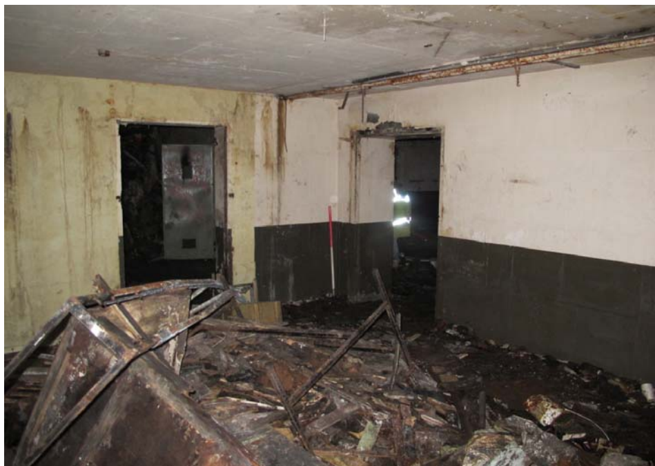
Figure 11: General shot of western room G3, showing the northern and eastern doorways. Looking northeast.
