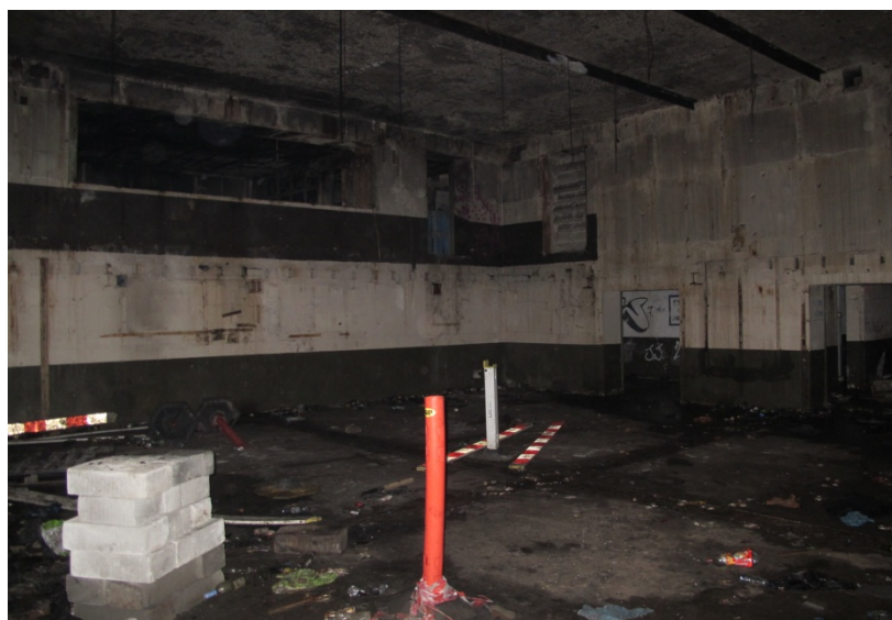
Figure 36: General shot of the main operations room showing the eastern end of corridor F4 terminating with an open doorway on the first floor. Looking northeast.
