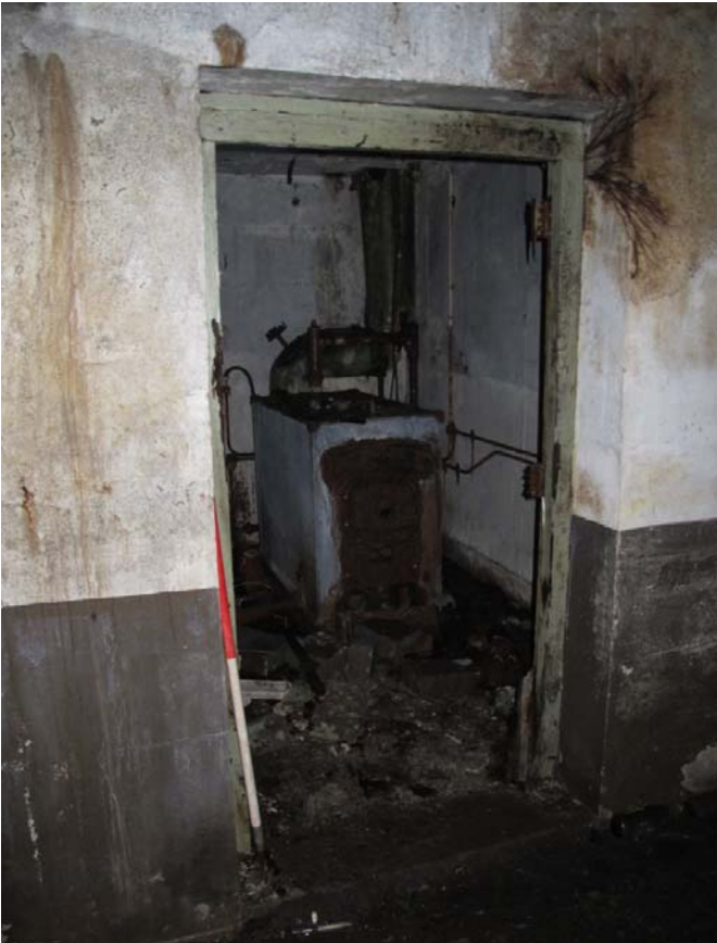
Figure 21: Shot of the northern doorway into the boiler room G11 from corridor G1. The boiler itself can be seen in the south-western corner of the room. Looking south.
