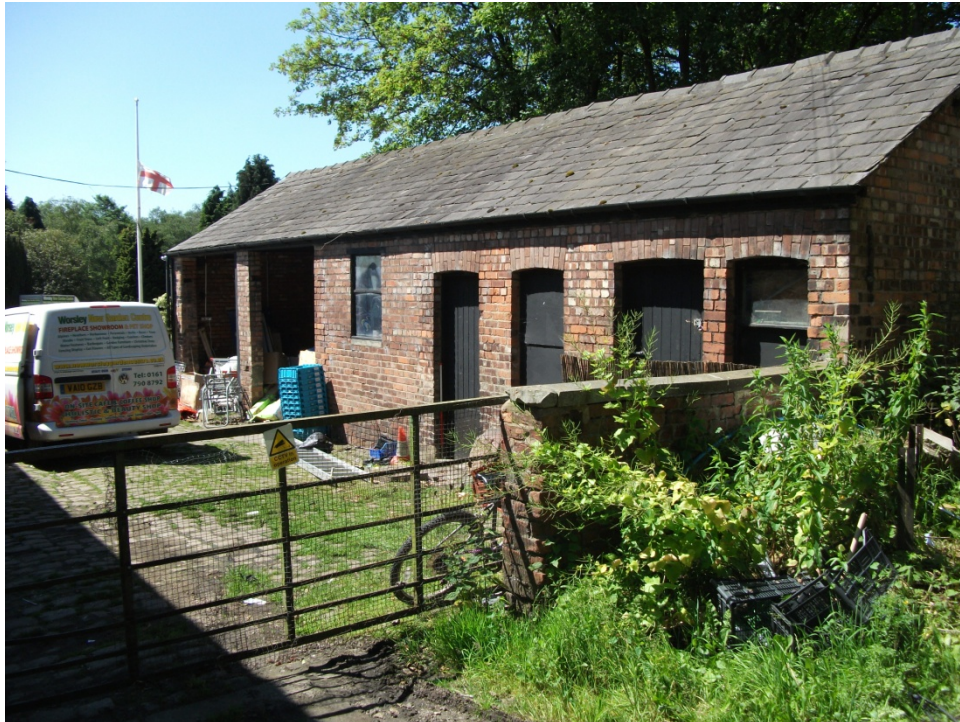
Fig. 7 - View of the stables eastern elevation. Looking SW
