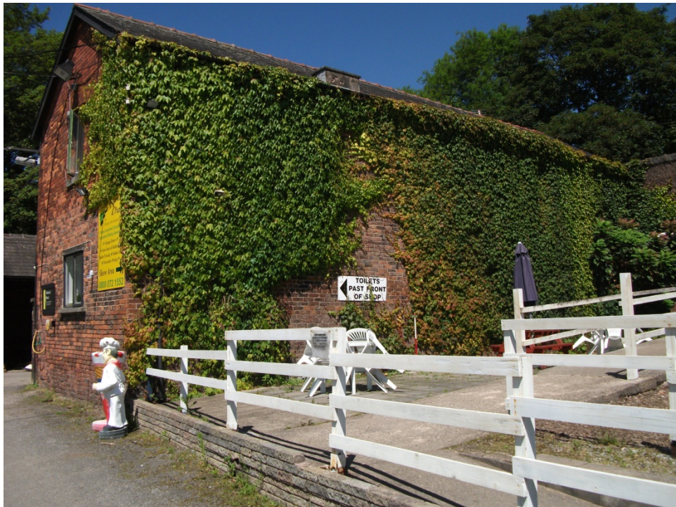
Fig. 14 - View of barns eastern elevation and southern gable end. Looking NW
