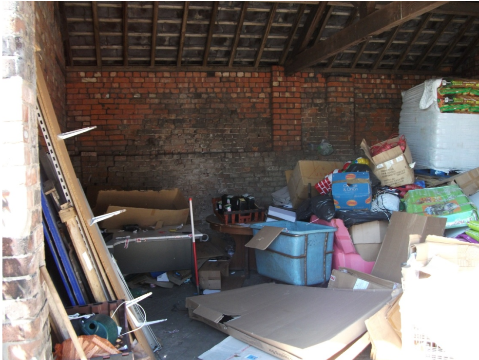
Fig. 11 – View of western wall in Western Stable. Looking W
