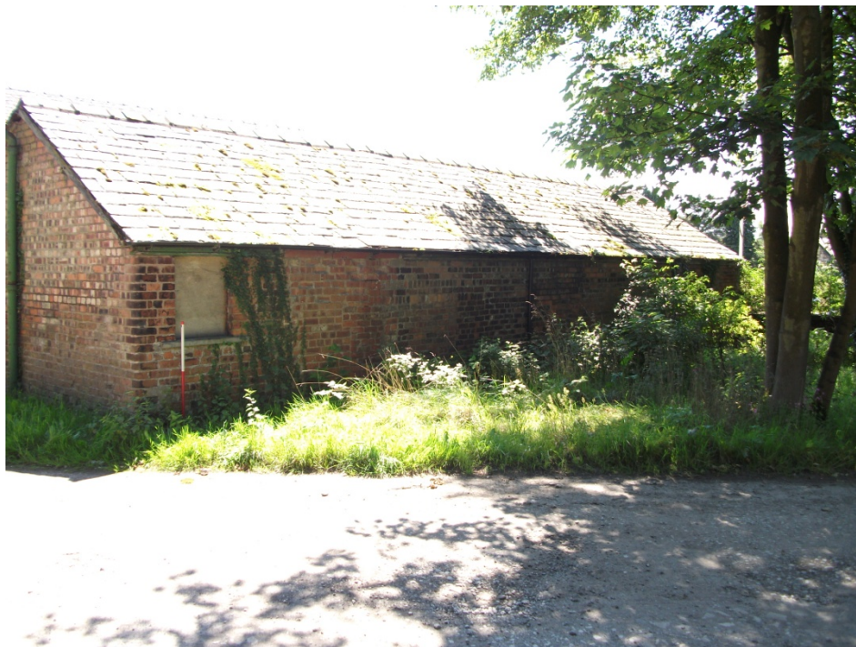
Fig. 8 - View of the Stables western elevation. Looking SE
