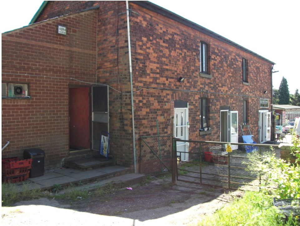
Fig. 13 - View of barns northern gable end and western elevation. Looking SE
